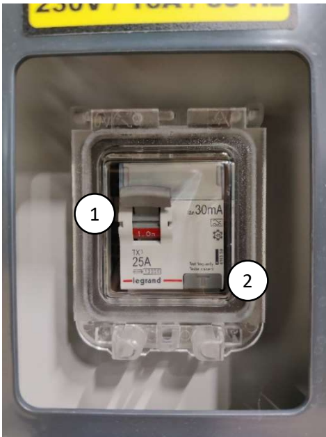
Figure 12. Residual current device
